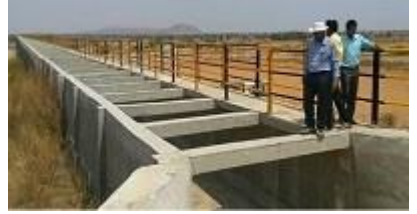
Aqueduct on Sonthi Main Canal
